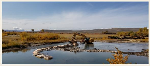
Photo: Using GPS technology, the contractor carefully places one big rock at a time to ensure the rock structure functions properly. This is a double cross vane structure. It will replace the temporary, cobble push-up dam that is constructed and washed out annually, adding sediment to the river.
